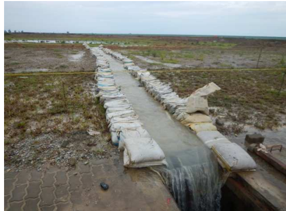
Tentative Drainage (to prevent soil erosion)
