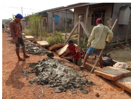
Photo 7-4 Drainage Cleaning
